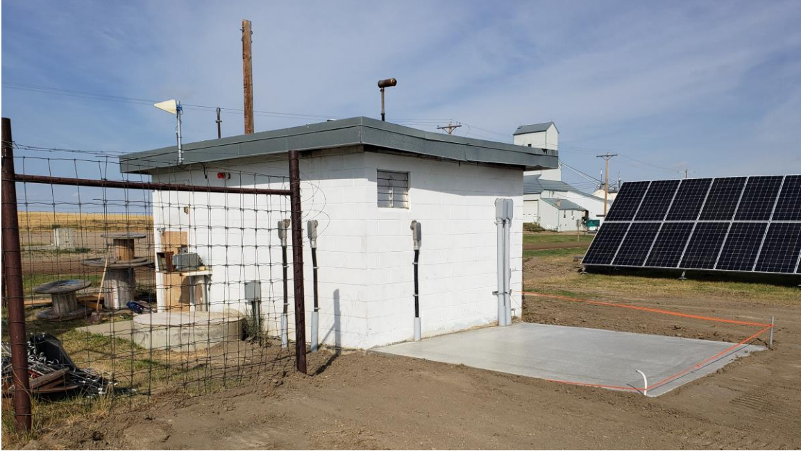
Lift Station extension
